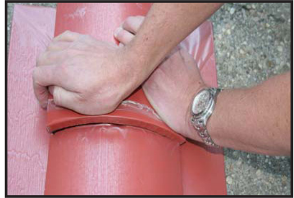
Step 4: With second hand push down to engage this tile on to the first tiles flange, some force will be required to POP this tile into place
