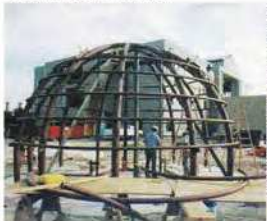
Left to Right: The dome of the Hinton Center was first fabricated on the ground and clad with solid decking, then covered with a membrane underlayment, and finally hoisted atop the rotunda. The final photo shows the special Berridge Compound Curved Tee-Panels being applied to the dome.
