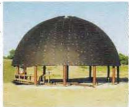
Left to Right: The dome of the Hinton Center was first fabricated on the ground and clad with solid decking, then covered with a membrane underlayment, and finally hoisted atop the rotunda. The final photo shows the special Berridge Compound Curved Tee-Panels being applied to the dome.
