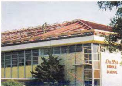
Fig. 1: Retrofit roof framing over old flat roofs.
