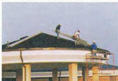
Fig. 4: Berridge Tapered Tee-Panels covered the circular port cochere.
