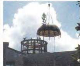
Left to Right: The dome of the Hinton Center was first fabricated on the ground and clad with solid decking, then covered with a membrane underlayment, and finally hoisted atop the rotunda. The final photo shows the special Berridge Compound Curved Tee-Panels being applied to the dome.
