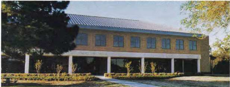
The Eula Mae Baugh Center, which houses a cafeteria and other student facilities, features a Berridge Zee-Lock standing seam roof.
