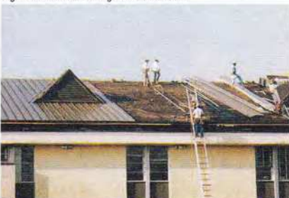
Fig. 3: Berridge Zee-Lock panels were installed over felt underlayment
