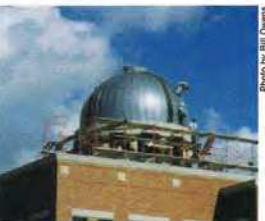
The Eula Mae Baugh Center, which houses a cafeteria and other student facilities, features a Berridge Zee-Lock standing seam roof.
