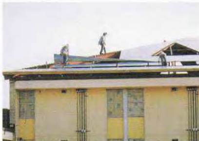
Fig. 2: Corrugated steel decking was applied over framing
