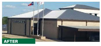
**Solution:** Berridge Vantage Point Retrofit Roof System provides a totally new design appearance, hides unsightly mechanical equipment and offers watertight integrity.
