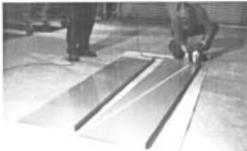
FIG. 2: MARK A CHALK LINE FOR THE DIAGONAL TAPER CUT....
