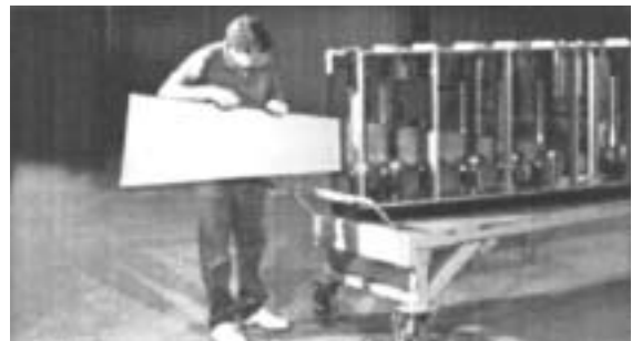
FIG. 5: EXERCISE CARE IN HANDLING LONG TAPERED PANELS
