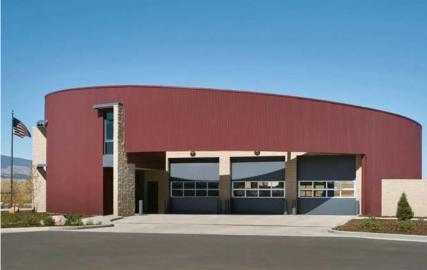
The Berridge S-Deck Panels are corrugated structural metal and can be installed horizontally or vertically with exposed fasteners. S-Deck may be curved making it ideal for use over covered walkways and shelters. This panel is available in two coverage options, two substrate options and is ideal for a variety of uses.
