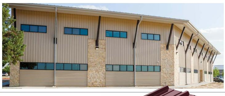
The Berridge "R" Panel is a wide, economical panel providing 36" of coverage for vertical or horizontal applications. Similar to the "M" Panel, this exposed fastener panel provides a different pattern option for a wide range of applications.
