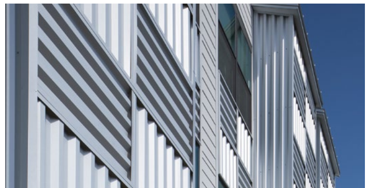
Pictured Above Project: NOBAY Village Architect: WMB-ROI Architecture General Contractor: RODDA Construction, Inc. Installing Contractor: CA Systems Color: Acrylic-Coated Galvalume®
