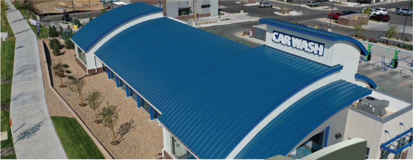
*The Berridge Zee-Lock Panel can be curved or tapered over solid sheathing or open framing making for limitless design possibilities.*
