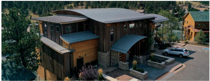
The Berridge Tee-Panel includes the patented vinyl weatherseal and the ability to be curved and/or tapered on-site, allowing for a custom installation.
