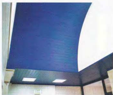
The atrium ceilings used Berridge Flush Seam Soffit Panels.
