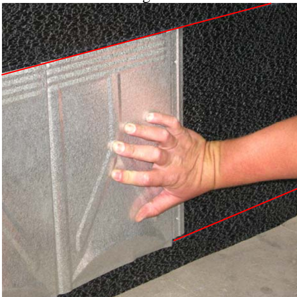
3. Keep top of shingle aligned with chalk line.
