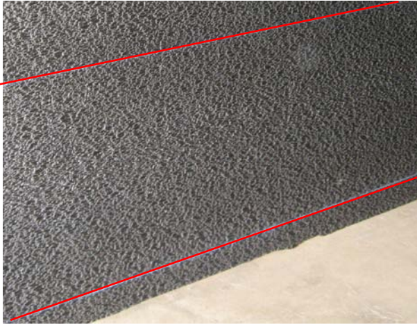
1. Strike chalk lines along the roof deck.
